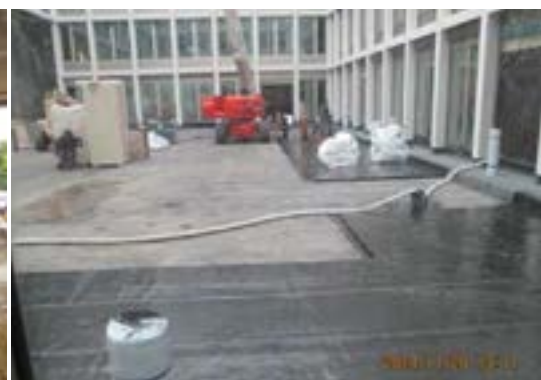
Courtyard, waterproofing works (20.11.2014)
